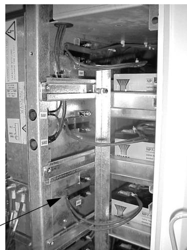
Check all battery connections to ensure that contact is established.
